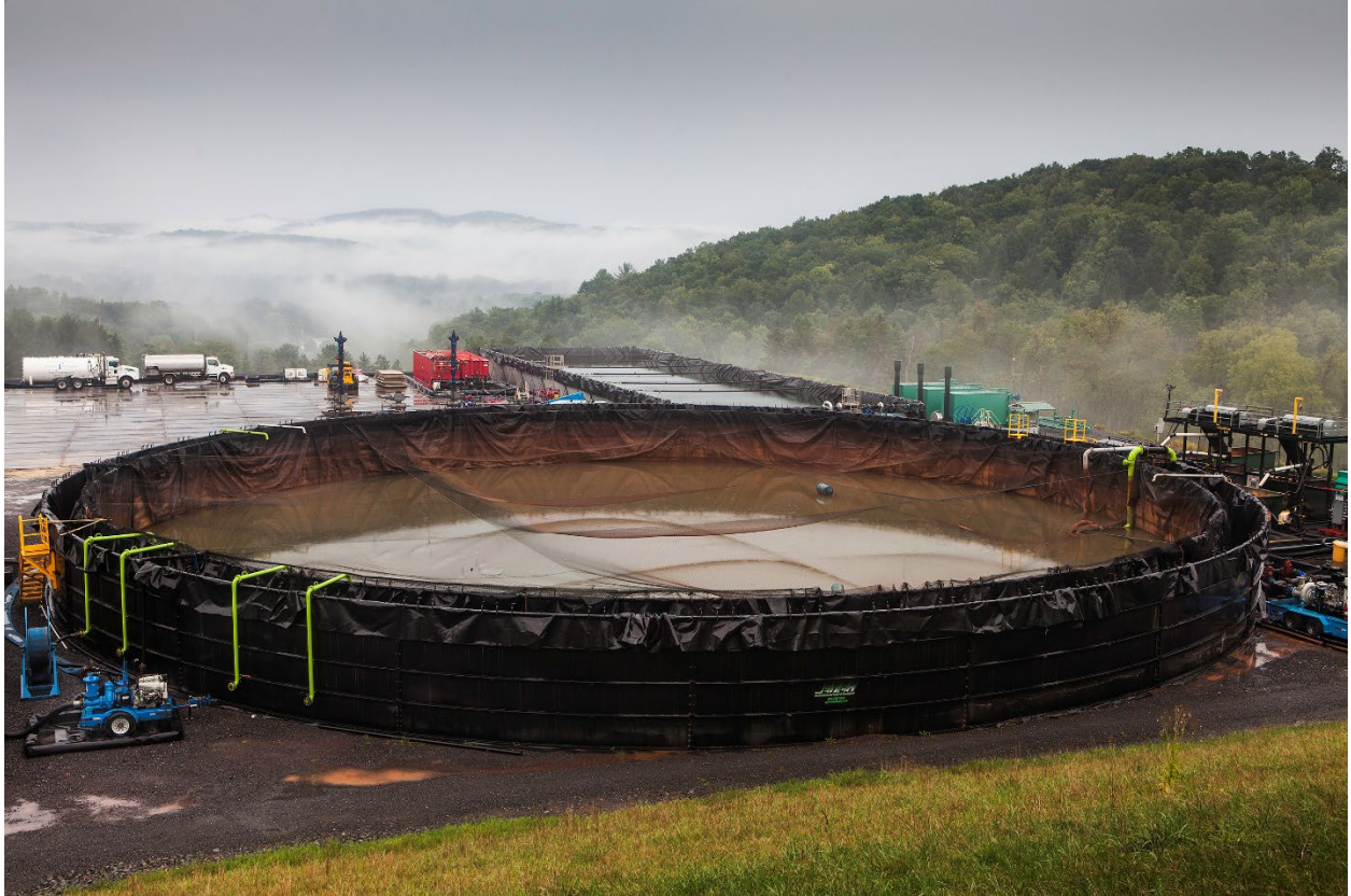
Figure 2. A large capacity fracking tank holds flowback water during a fracking operation at the Inflection Energy well pad on Yeagle Road in Eldred Township, Lycoming County, Pennsylvania. The Department of Environmental Protection has cited Inflection Energy for repeated violations at this site, including the company's failure to properly cement gas wells, and for spilling approximately 63,000 gallons of flow-back fluid, which discharged into a nearby tributary to Loyalsock Creek. All of the nearby residents rely on private water wells for their water supply. September 18, 2016.
