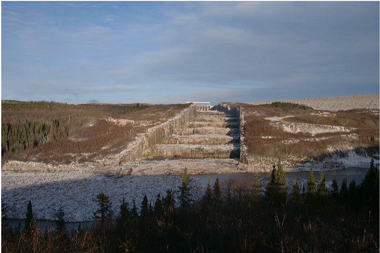
Figure 2: The spillway at the Robert-Bourassa hydroelectric complex, in northern Québec [The Staircase of the Giants]. Photo credit: Peter Van den Bossche, Wikimedia Commons. https://commons.wikimedia.org/wiki/File:Staircase_of_the_giants-2.jpg
